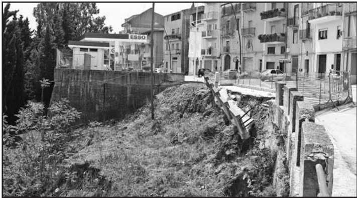
La frana in via Marsala
